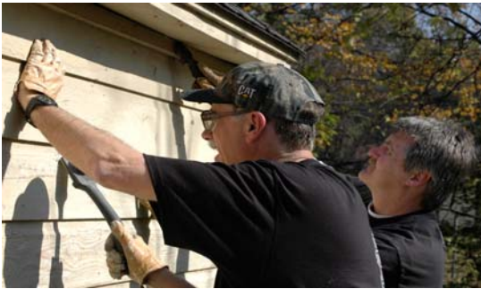
Roger DeShaies and John Peebles of St. John's Episcopal scrape and prepare the siding of this garage for painting.
