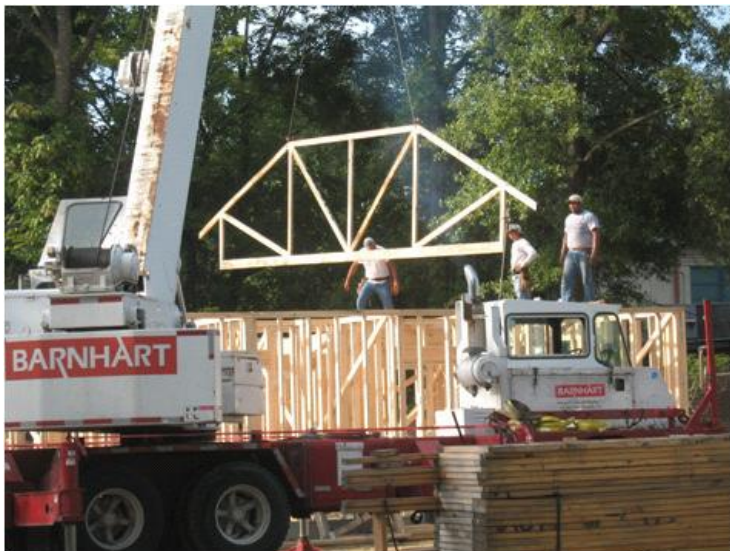
Setting Roof Trusses in early October, 2013
